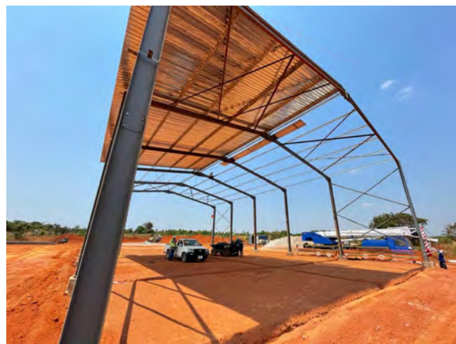
Recently constructed workshop
