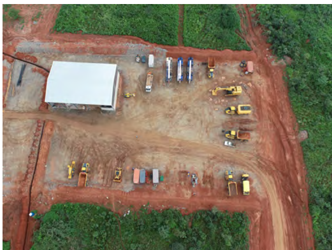
Aerial shot of Mimbula site, showing build workshop and equipment
